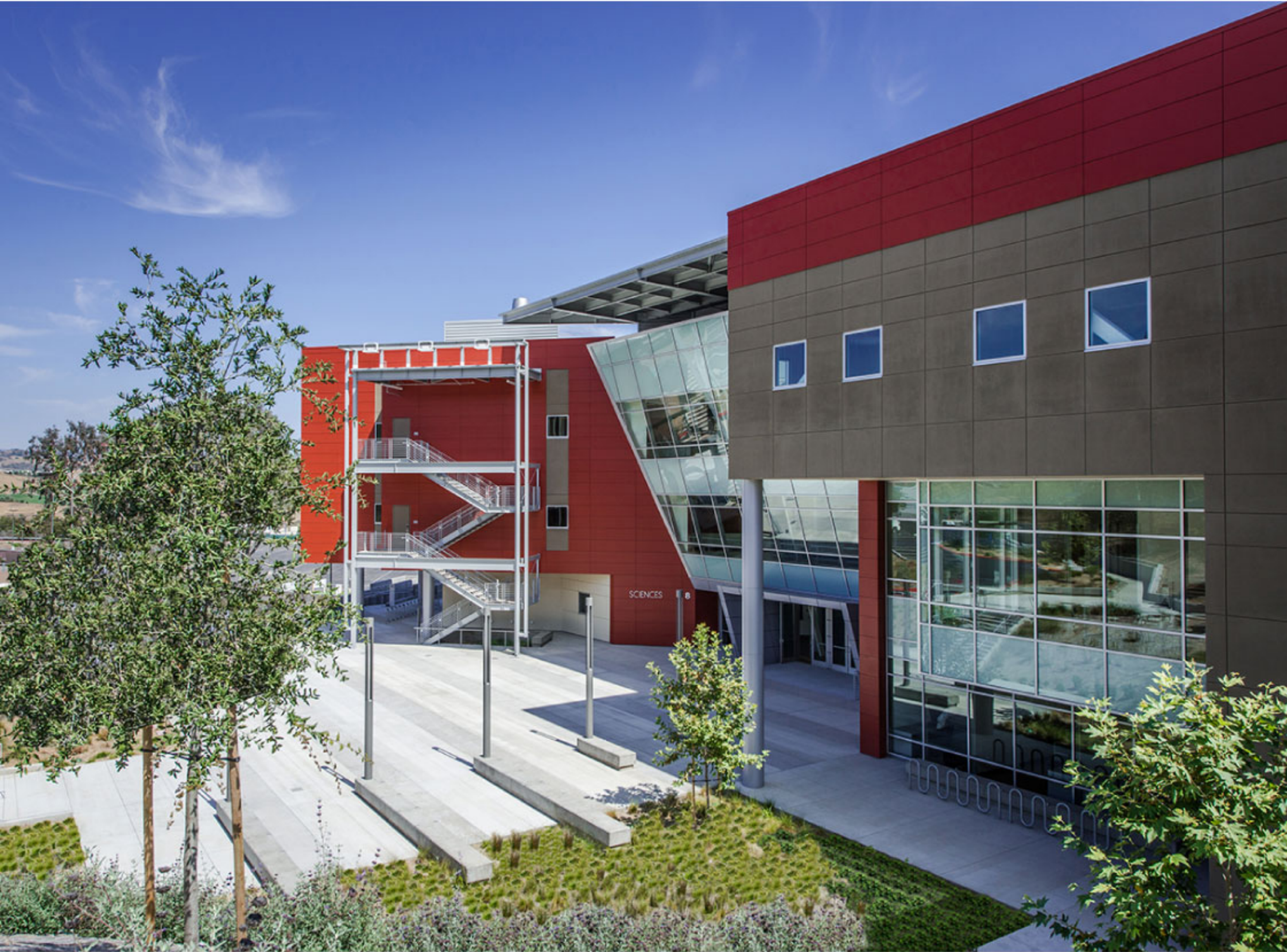
EXTERIOR VIEW NORTH FACADE/MAIN ENTRY
