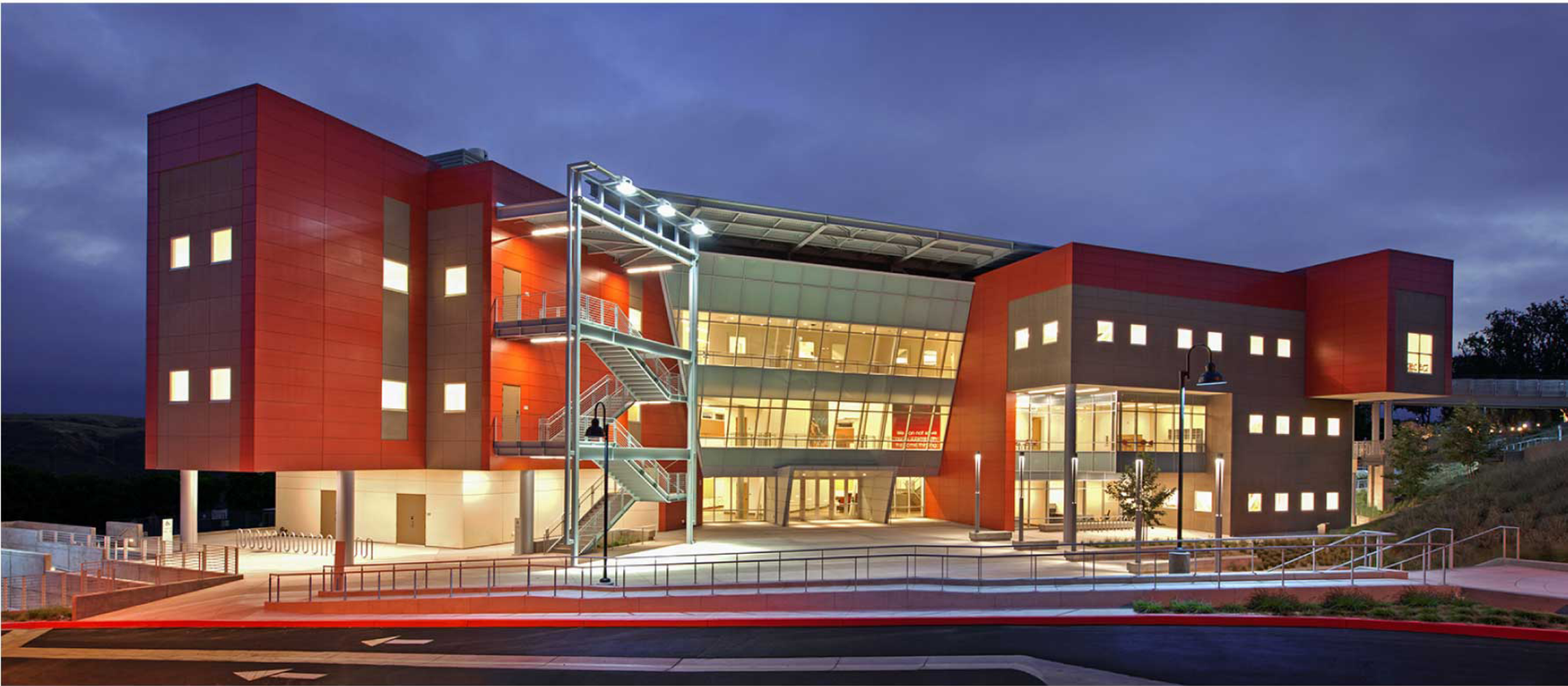
SADDLEBACK COLLEGE SCIENCE BUILDING SOUTH ORANGE COUNTY COMMUNITY COLLEGE DISTRICT
