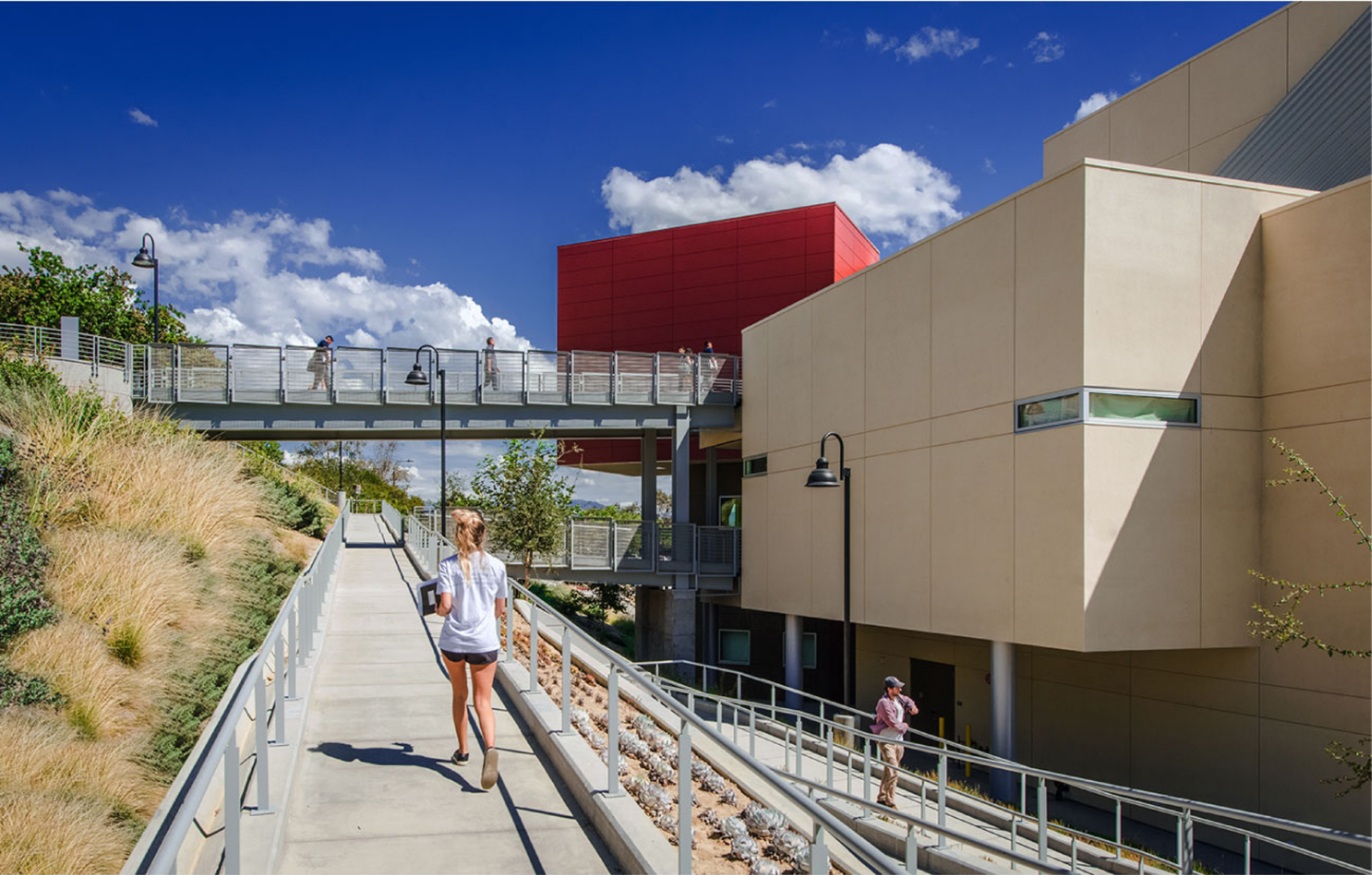
EXTERIOR ACCESSIBLE RAMP SYSTEM WEST FACADE
